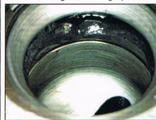
Magnified view of o-ring damage.
